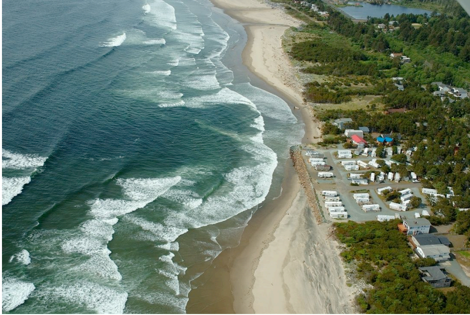
Figure 6.12 Ongoing shoreline retreat over the past decade in the Rockaway cell and localized hotspot erosion effects have resulted in substantial sections of the shore having to be rip-rapped in order to safeguard property. SLR expected over the next century and enhanced storms will almost certainly increase the risk of failure of such structures and the potential loss of homes and important infrastructure backing the beach.(Photo courtesy of Mr. Don Best, 2009.)
